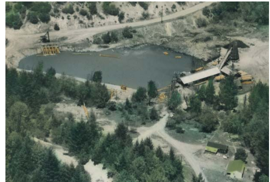
Southwick sawmill north of Willits California. Harold's house and sheds are in the foreground
