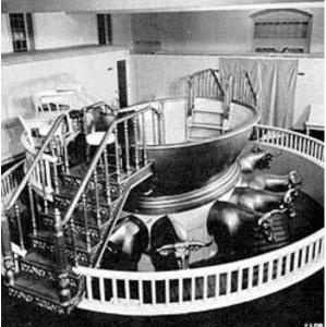
rail and then by special wagons. The parts were taken directly into the temple basement, where Nathan bolted and welded the font together. The temple was not finished and ready for dedication until April 1877.
