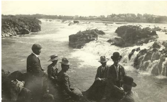
Before Idaho Falls Temple built and dedicated 1940-1945
